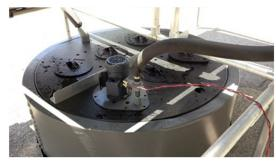
Storage Tank used as primary rack ballast resulting in no roof assembly or membrane Penetrations.
